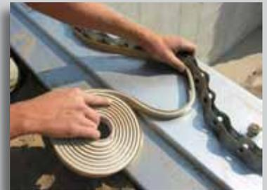
Mastic between all panel joints and foam sealer at the base provide a protective barrier against moisture and wind.
